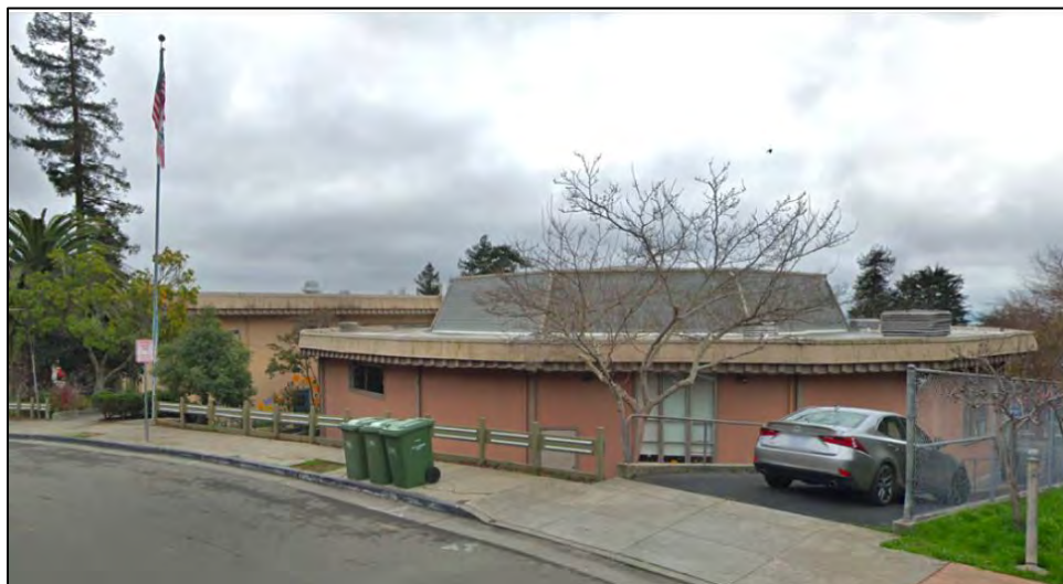
Figure 9: Oxford Elementary School (Source: Alternatives Analysis).
